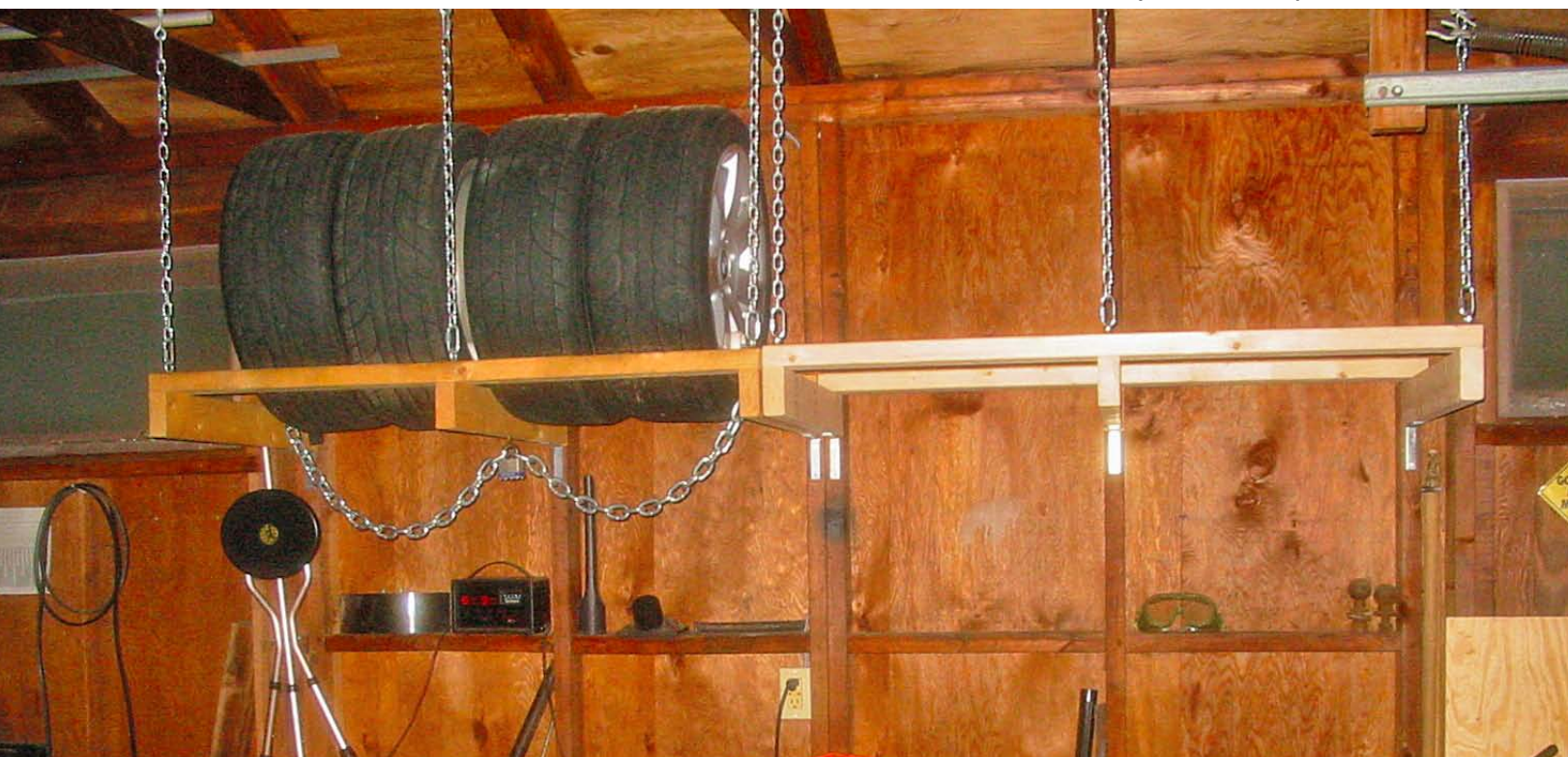
Photo 1: The completed tire rack is a sturdy storage solution.
